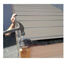
Step 22: Repeat above step through the rib at the opposite end of the top plates. Screw off the sheets (1 Screw per rib, per top plate)
