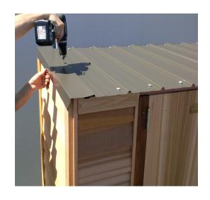
Step 31: Using 3 rivets, rivet ends of spouting to barges and rivet 1 rivet into roof sheet.
