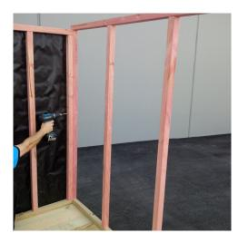
Step 8: Select remaining panels, predrill and screw together as shown.
