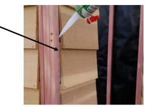
Step 11: Nail 15 x 17mm beads on front corners and beside doorway as shown, using 4 x 50mm stainless steel beading nails, per bead. Ensure top is flush with top plate.
