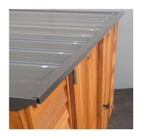
Step 32: Rivet ridge flashing to barges and roof sheets as above.
