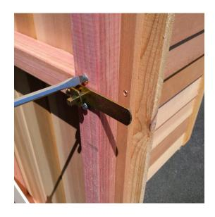
Step 29: Attach Cedar door blocks to both front wall panels, hard underneath roof.
