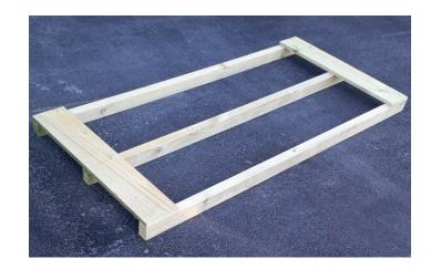
Step 2: Lay out remaining floor boards. Measure diagonals to ensure measurements are equal (i.e. floor is square). Rip down last floor board to suit gap, and nail off floor with 50mm flooring nails (2 nails per Joist, per board).
