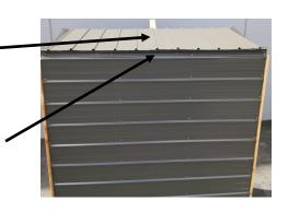
Step 21: Screw the first sheet with a 50mm roofing screw with washer. Screw though the rib of sheet into back wall top plate.
