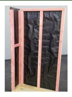
Step 5: Using a 6.5mm drill bit, predrill stud then screw wall panels together using 75mm tek screws (3 per join), ensuring end wall panels are inside side wall panels as per wall plan.
