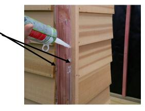
Step 13:Nail corner clashing's onto corners as shown, using 4 x 50mm stainless steel beading nails, per bead. Ensure top is flush with back and top plates.
