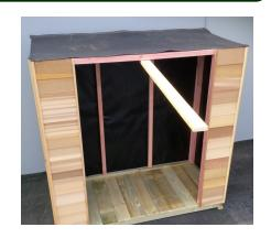
Step 20: Rivet the two roof sheets together, one rivet through the centre rib.
