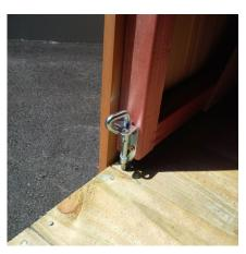
Step 27: Fasten Top padbolt as per above steps. Drill 10mm hole into underside of top plate.
