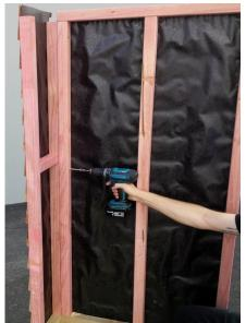
Step 6: Stand back wall frame ensuring angle on top plate is sloping towards the front.
