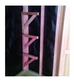
Step 33: Screw plywood shelves to brackets with 40mm screws, (6 per shelf).
